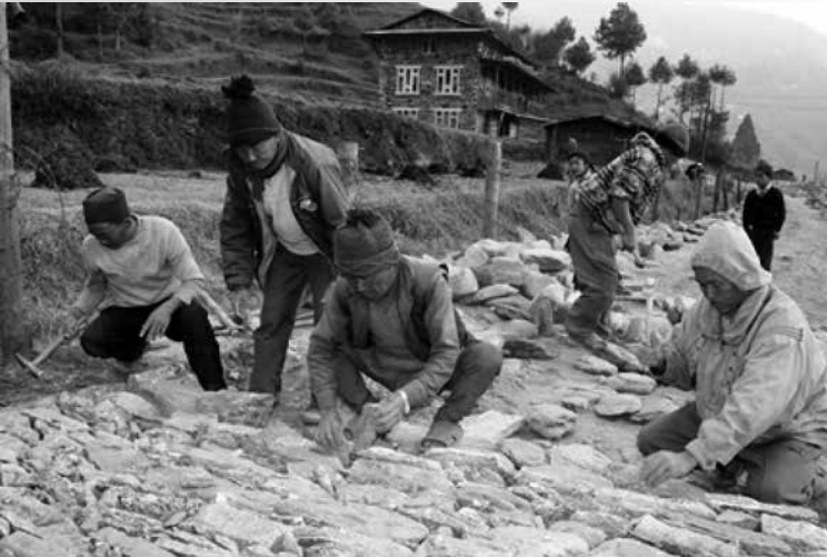
Figure: Green road construction
