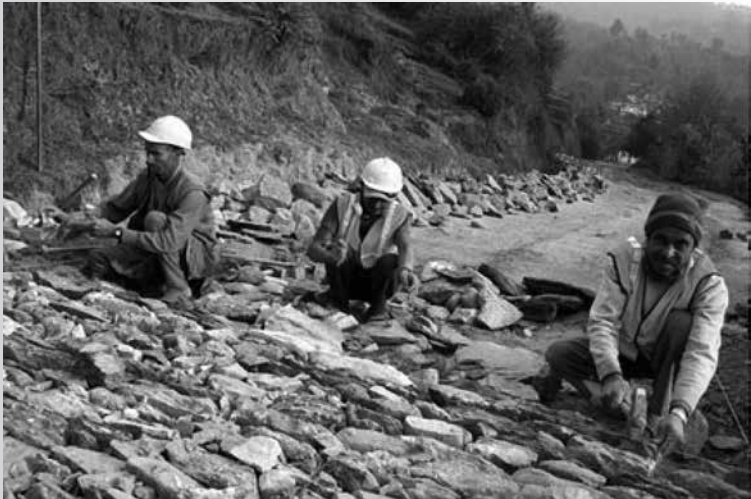
Figure: Green road construction
