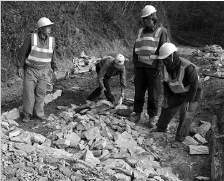
Figure: Green road construction
